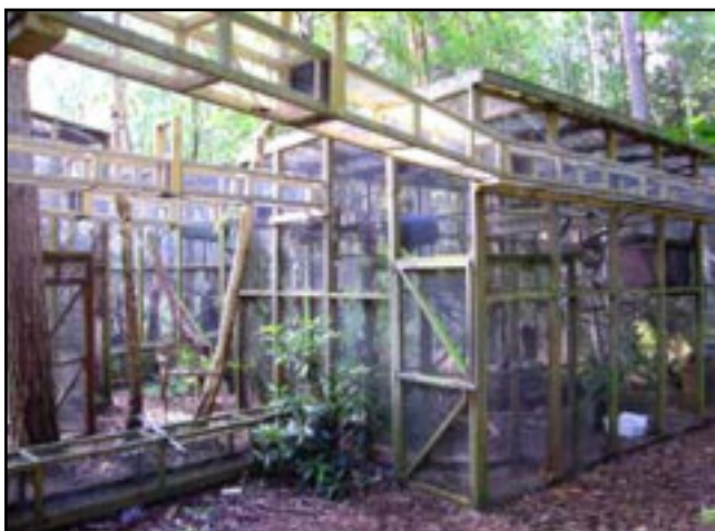
Tunnel system surrounding the enclosures
